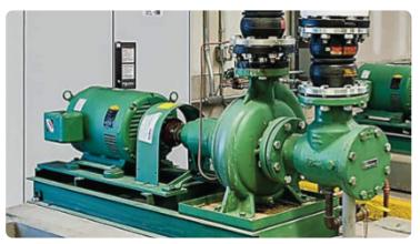
Misalignment is critical in direct coupled machines (with coupling)
